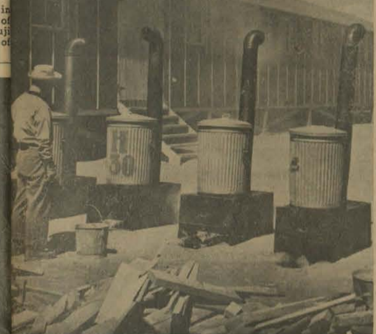
When the first family contingent arrived on April 1, 1942, the first dishwashers didn't just turn the handle on a faucet for their hot water. Manzanar was still under construction and boilers had not been installed so the phrase, "barest necessities of life" held much meaning for the pioneer evacuees. Water for mess hall use was heated on these wood burning Army field stoves.
