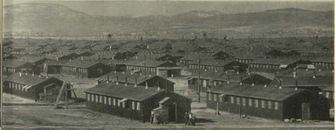
Barracks for Japanese are placed in rows like marching soldiers. Every one, tar-papered from rooftop to baseboard, is just like all the rest. Each chimney marks an apartment. Inside the
