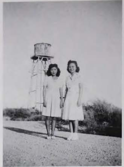
Miyo Higashi & Erma Okuda in front of water tower
