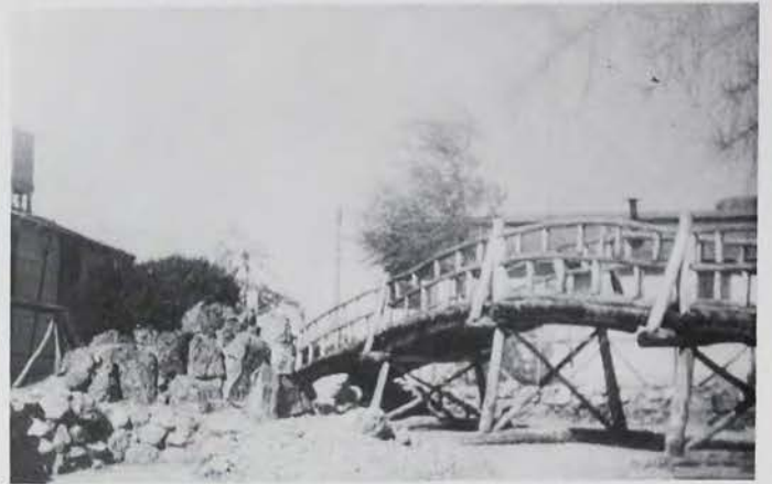
Bridge in back of Administration Building
