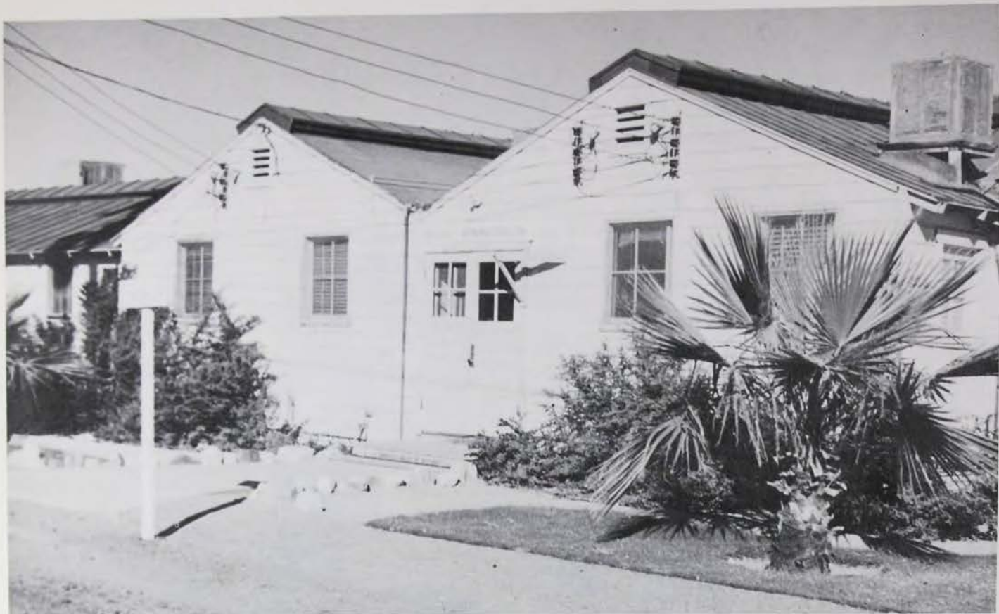
Main entrance to Administration Center
