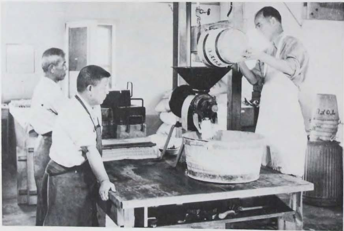
Tofu factory: funyu press - extract funyu from cooked and ground soy beans
