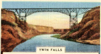
TWIN FALLS JEROME BRIDGE, SNAKE RIVER, 476 FT. HIGH
