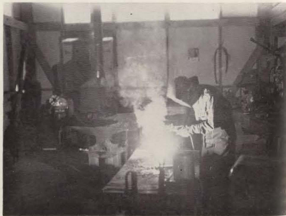
Welder at work.
