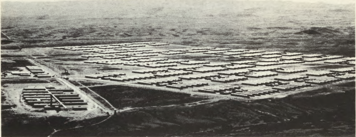
Detention camps were usually located in lonely and bleak areas. This is Heart Mountain, Wyoming, camp which held more than 10,000 persons.
