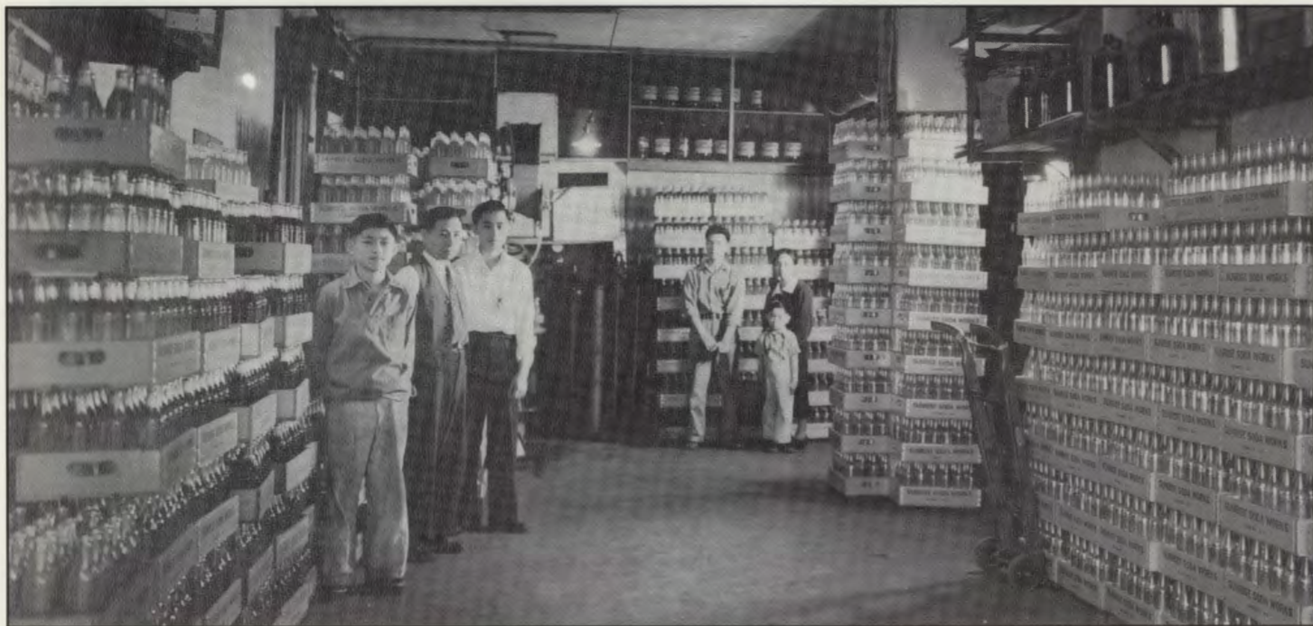
Mayeda Family's Sunrise Soda Works
