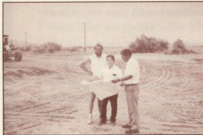
July 28, '92, "Hutch" Hutchinson, Ted and Ron Moore site preparation begins.
