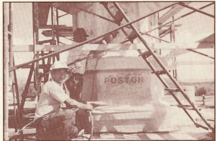
Ted Kobata and Mas Sunahara washing off the concrete retardant
