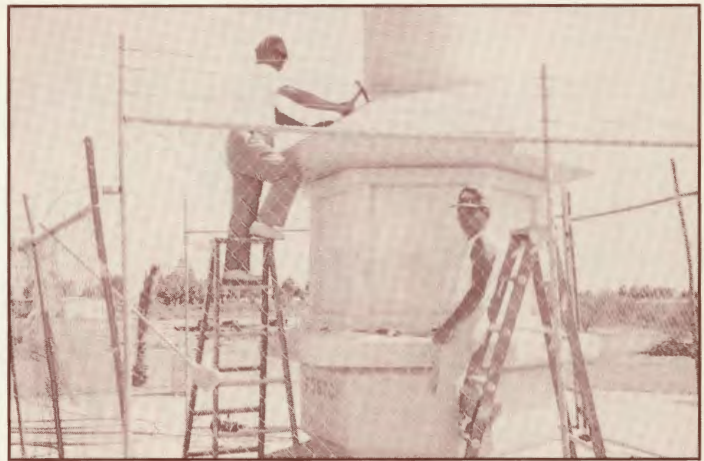
Two Georges, Oki and Yomogida, put finishing touches with chipping hammers.
