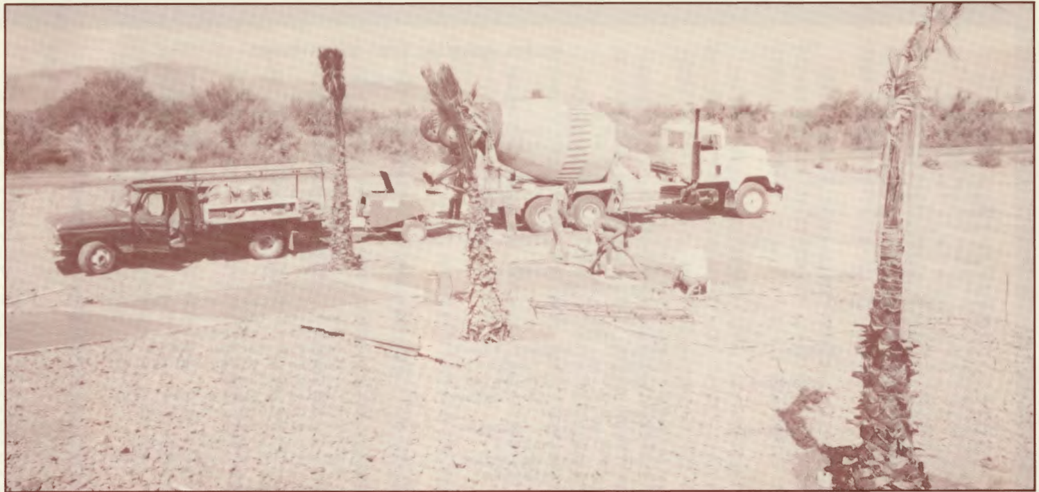
The final concrete pour of the walkway, September 18, 1992.
