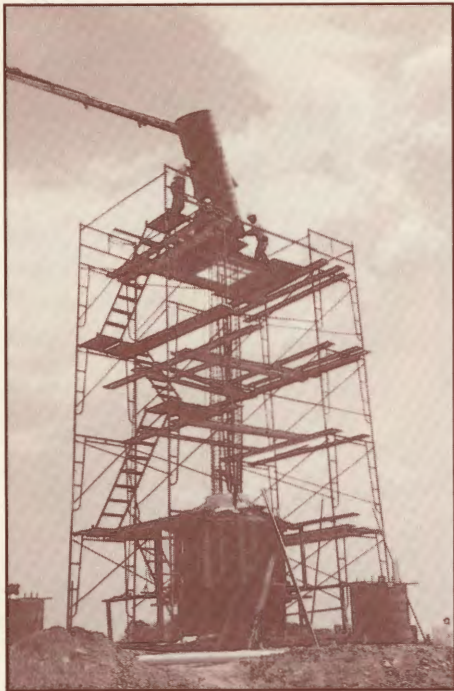
Installation of the 3 ft. diameter sauna tube form.
