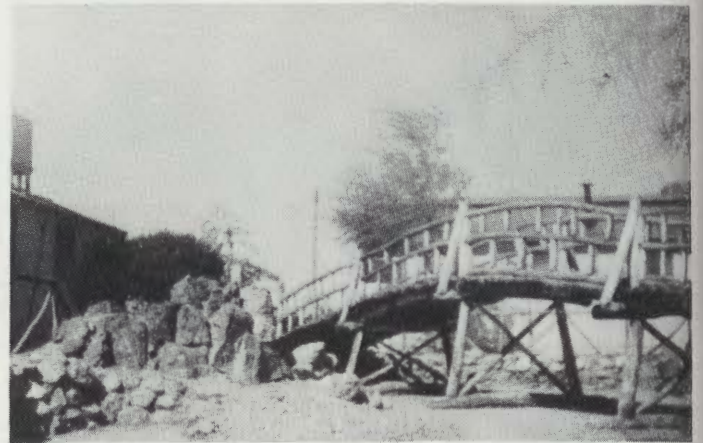
Bridge in back of Administration Building
