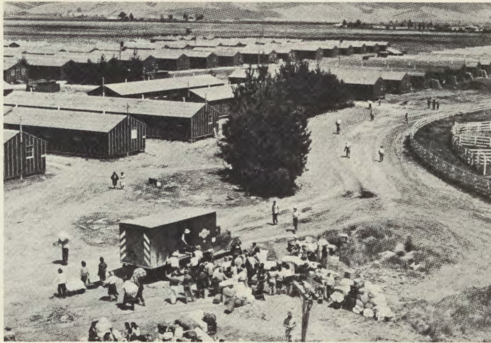
SALINAS ASSEMBLY CENTER (RODEO GROUNDS), 1942
