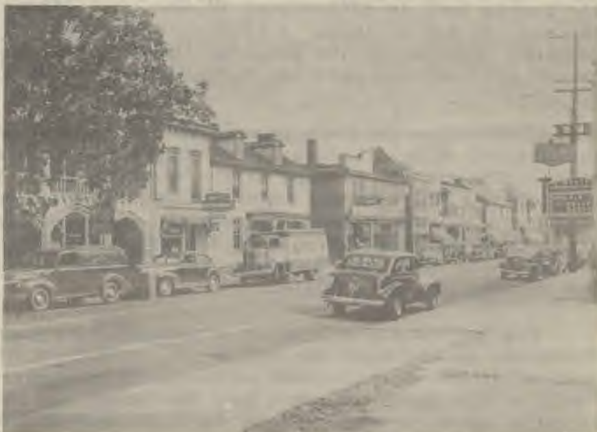
Main Street in one of Delaware's small towns, trade and market centers for farm areas nearby.
