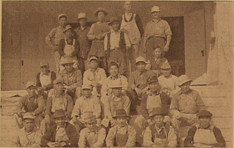
Above is pictured the skeleton crew composed of K. Ishimitsu and his 20-man carpenter crew which has been working on the gym-auditorium construction since the building's beginning days.
