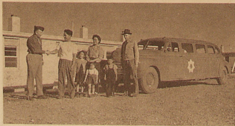
Pictured above is the family of Kaz Kimura first evacuee to arrive at the Sioux Ordnance Depot at Sidney, Nebraska. He is shown being greeted by one of the officers at the plant. This photo shows the exterior appearance of the housing project at Ordville.
