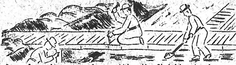
Several workers are shown putting the finishing touches on a bridge over a ditch in the above sketch.
