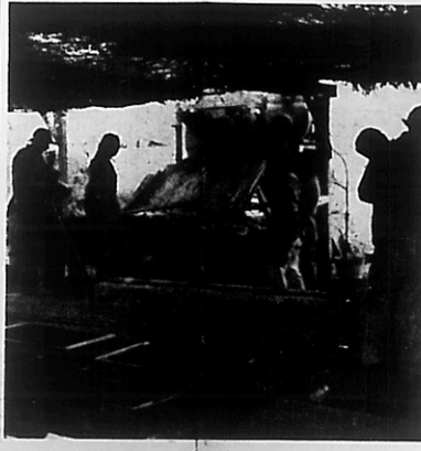
Women as well as men help make adobe bricks which are being used for the construction of public school buildings at the Colorado River War Relocation Center. The above picture was taken during the busiest day in the adobe production work.
