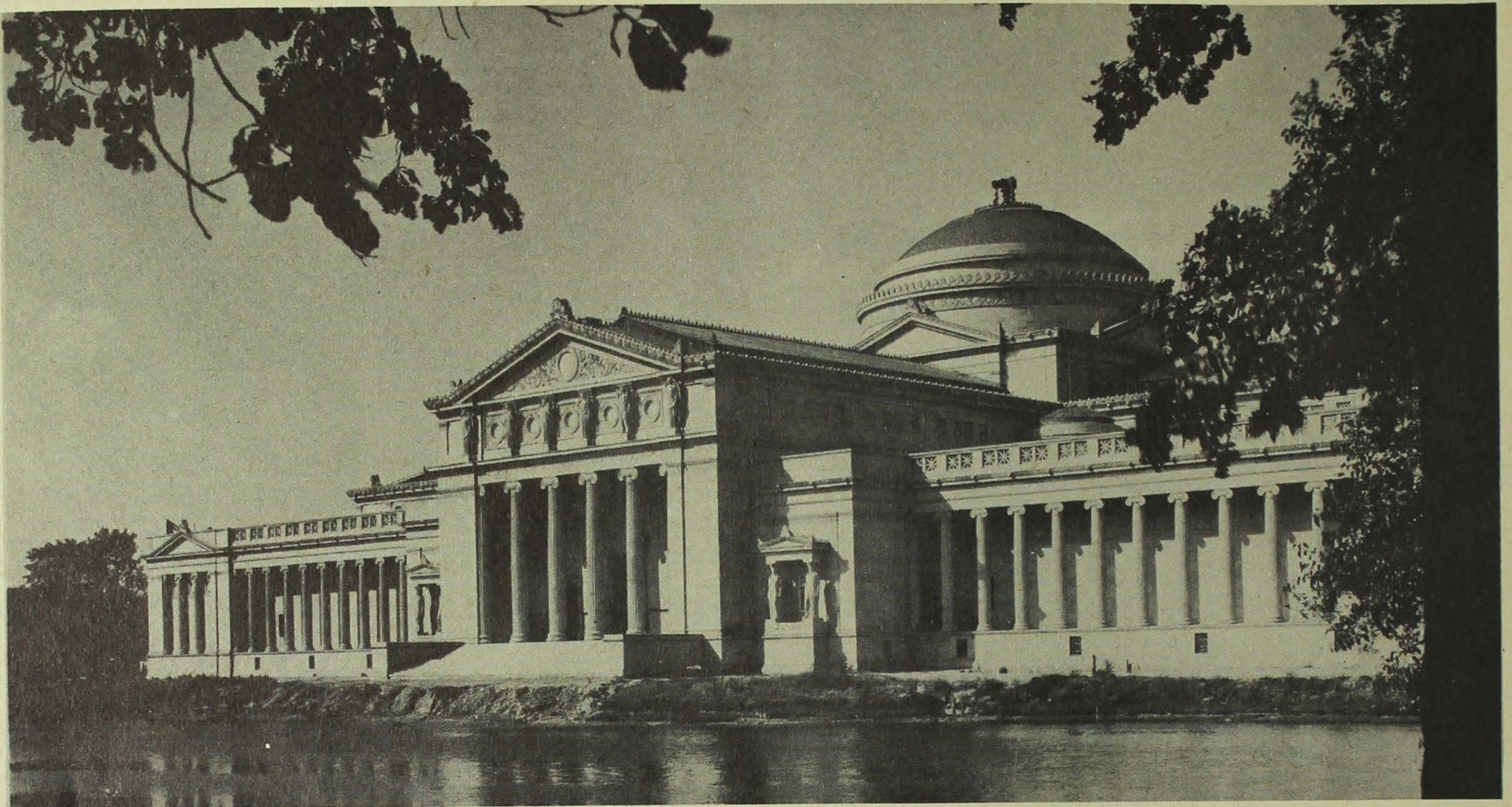
Museum of Science and Industry in Jackson Park One of the nation's most beautiful architectural achievements.
