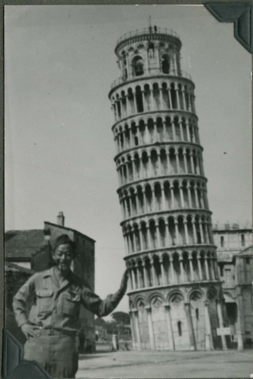
Leaning Tower of PISA
