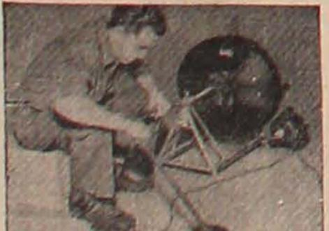
We have recently installed the most modern type of Electric Sewer Cleaning Equipment and are now able to handle a much greater volume of this work, including roots and other serious stoppage.
