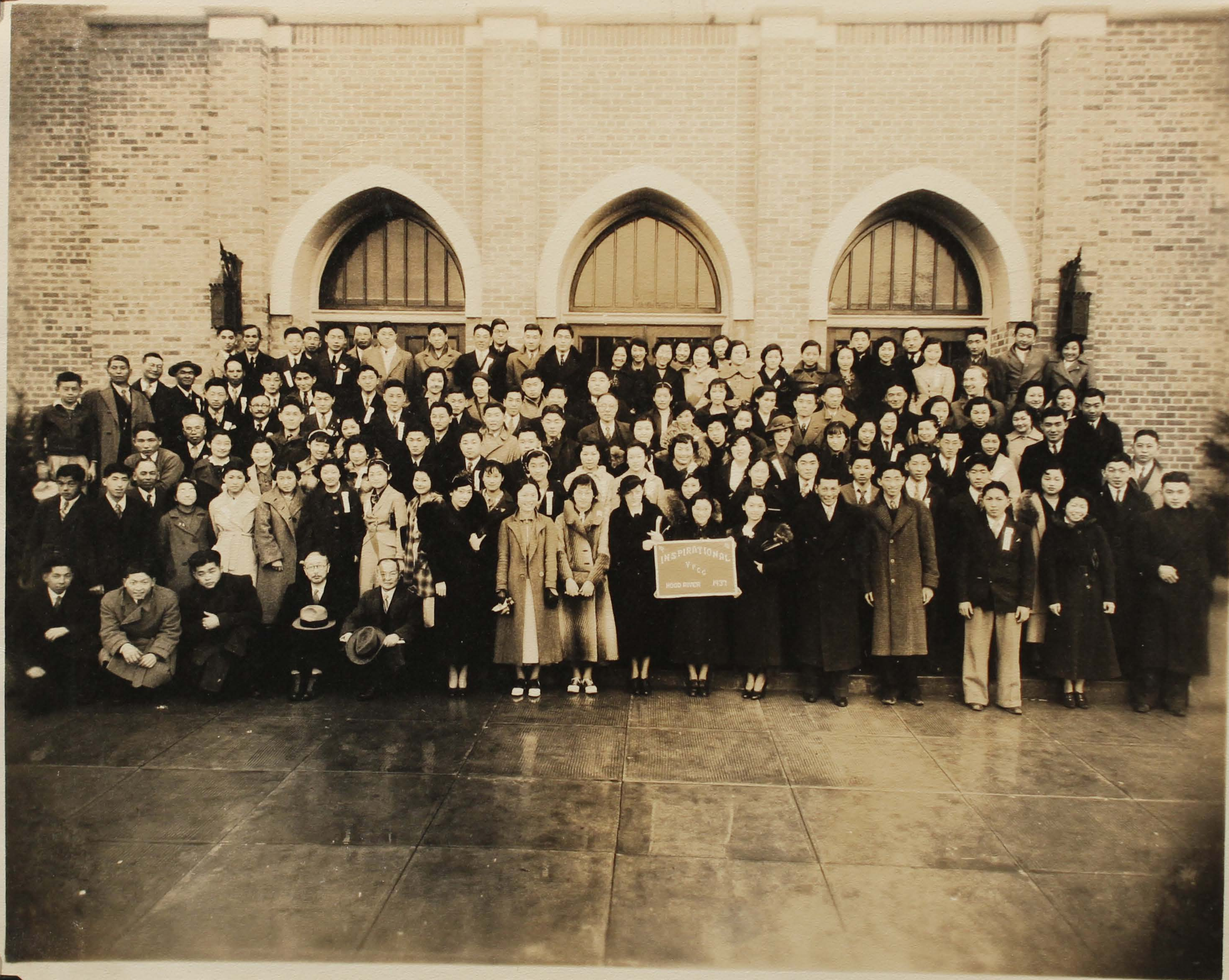
FRONT OF HOOD RIVER HIGH SCHOOL
