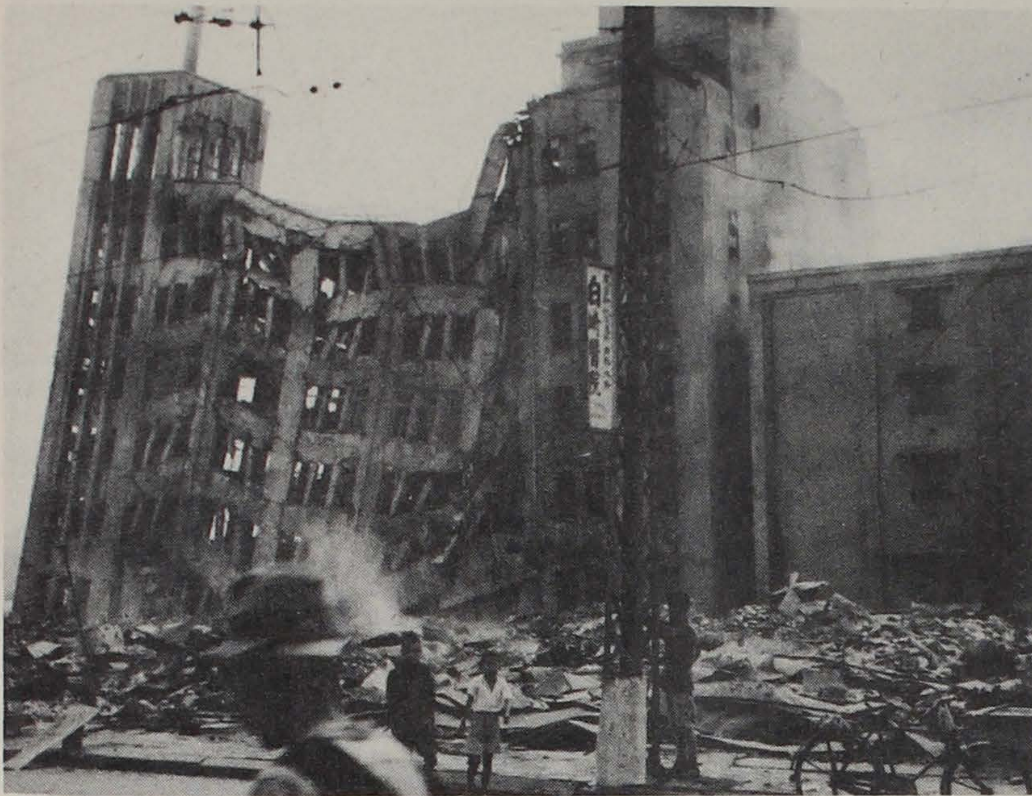
HUGE DAIWA BUILDING lists drunkenly at 5:14 p.m. Soon gutted by fire, the building is smouldering rubble by morning.
