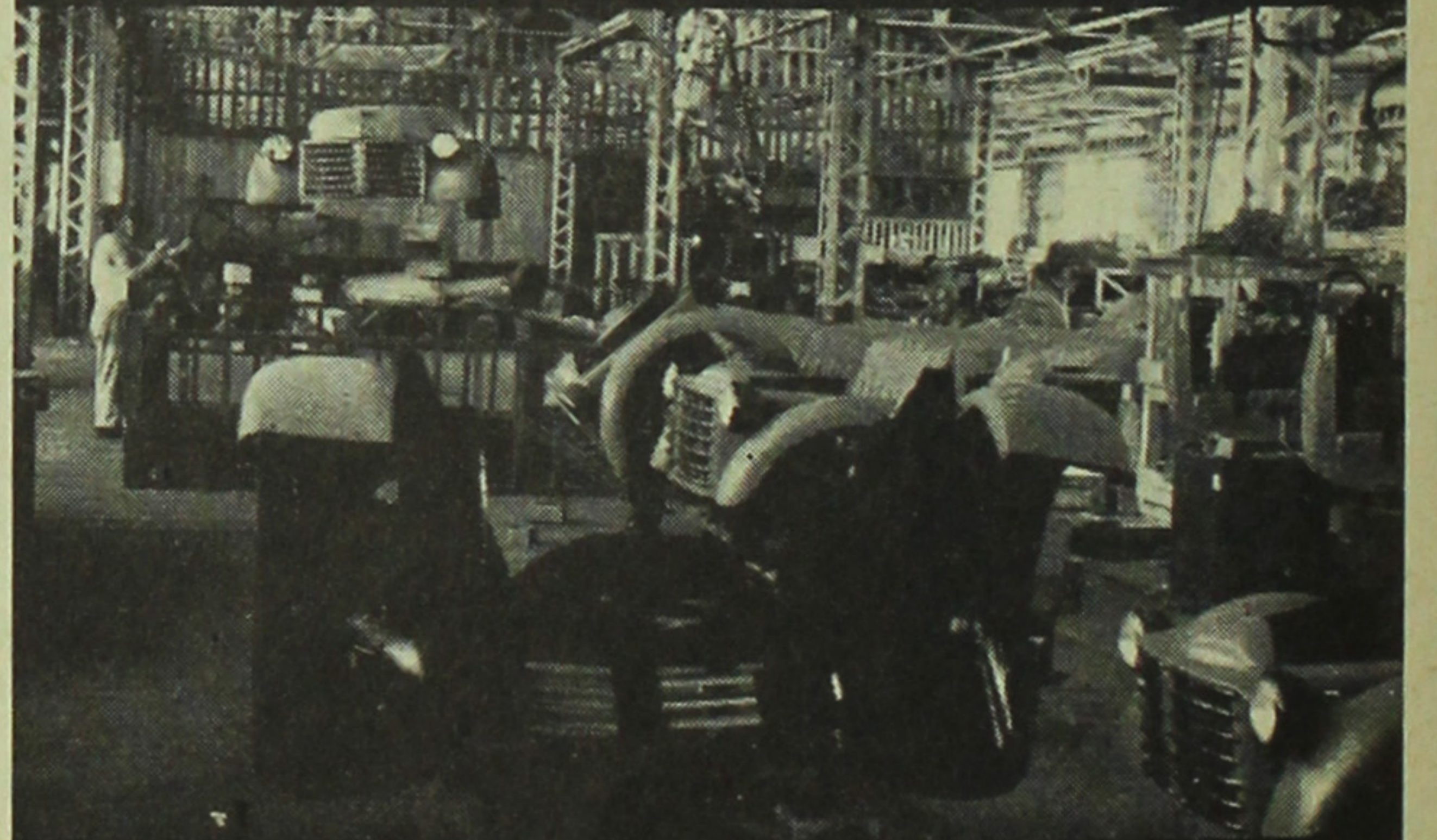
Assembly plant of Toyota Car Co.
