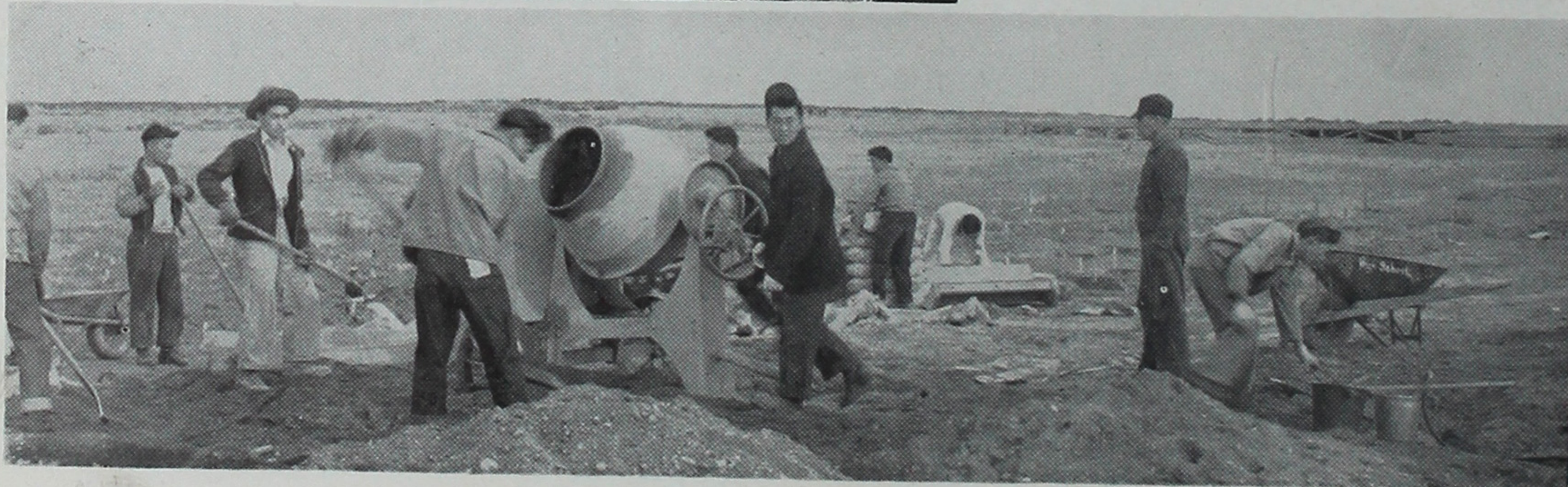
● Workshop Construction Crew
