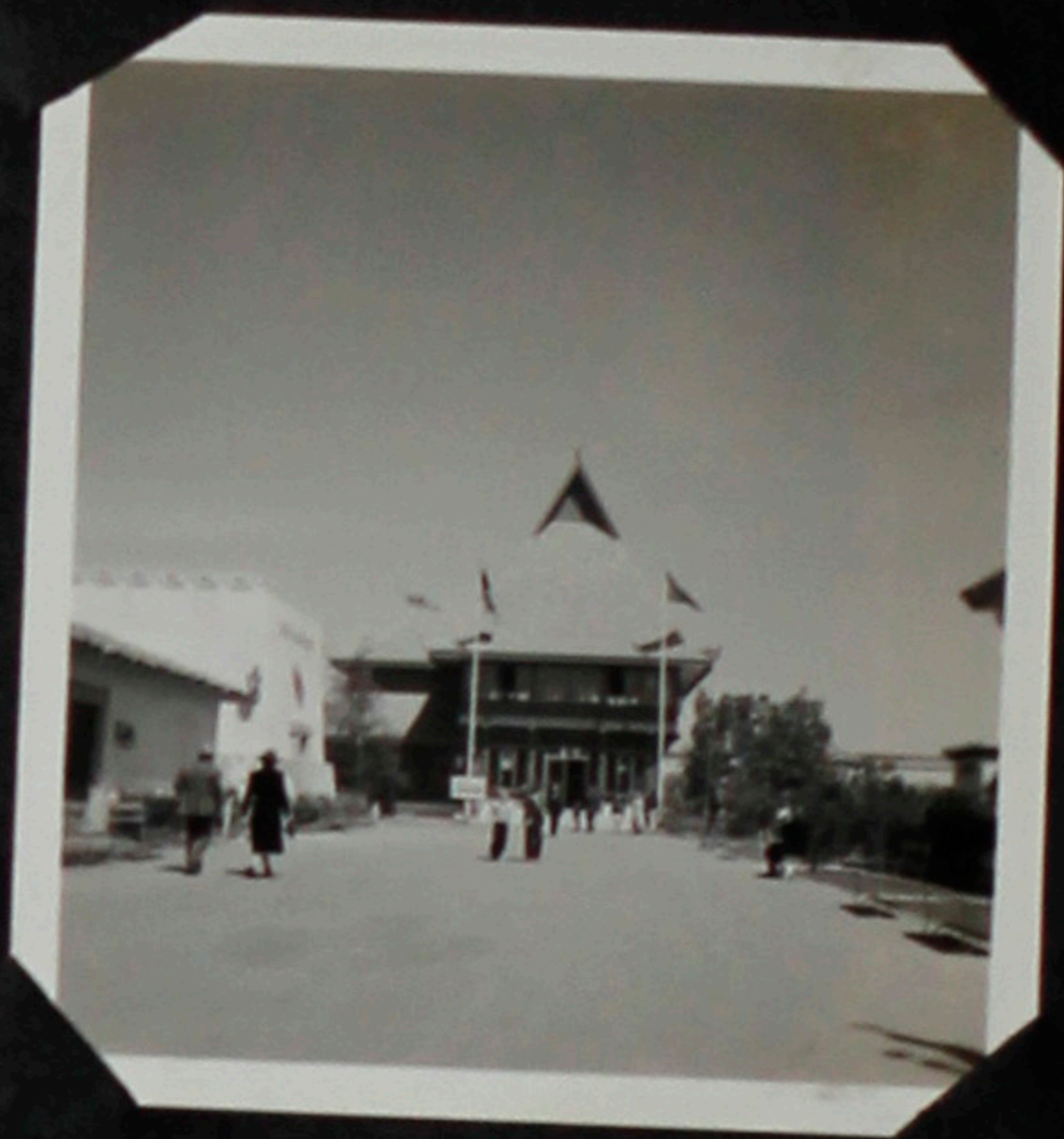
State of Johore Pavilion
