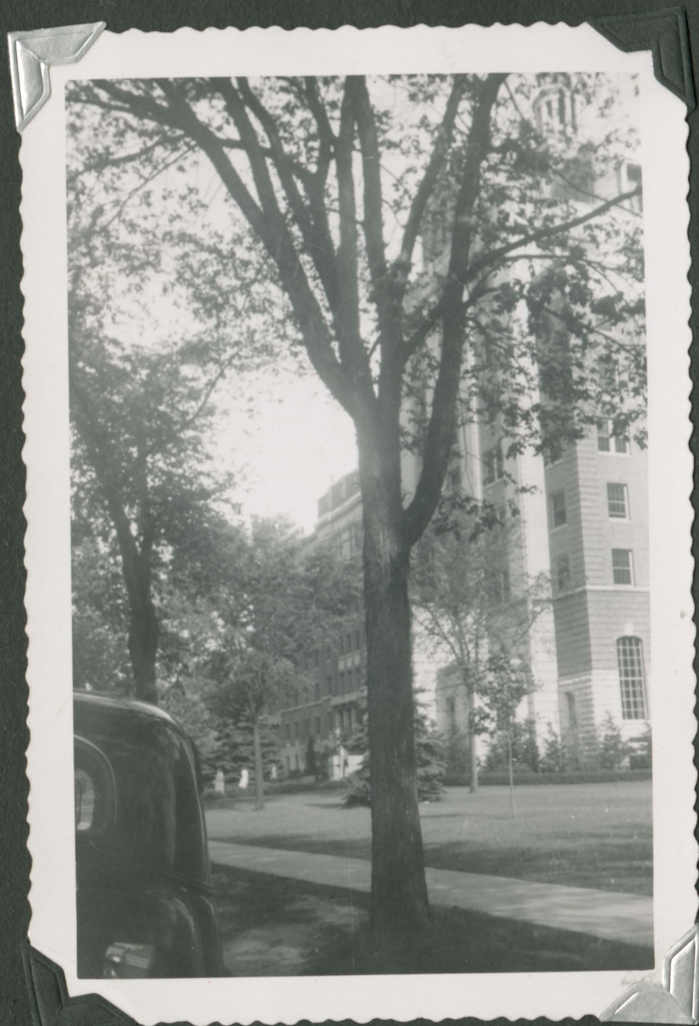
Mayo Hospital Building
