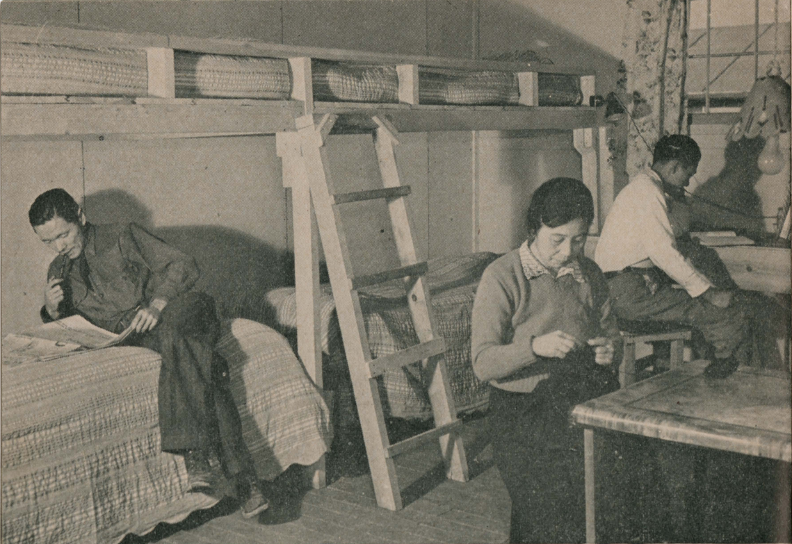
Improvements in family living quarters are made by the evacuees themselves from scrap materials.
