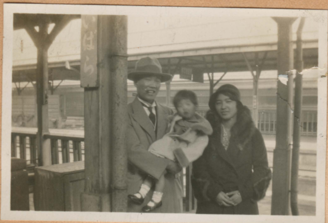
at Maebara Station on way to Goshu
