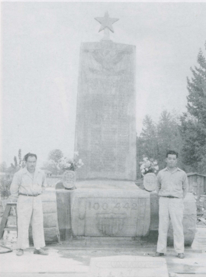
MONUMENT BUILDERS —Kaneo Fujioka (left) and Kay Horisawa (right) engineered and constructed this concrete monument in 1945.
