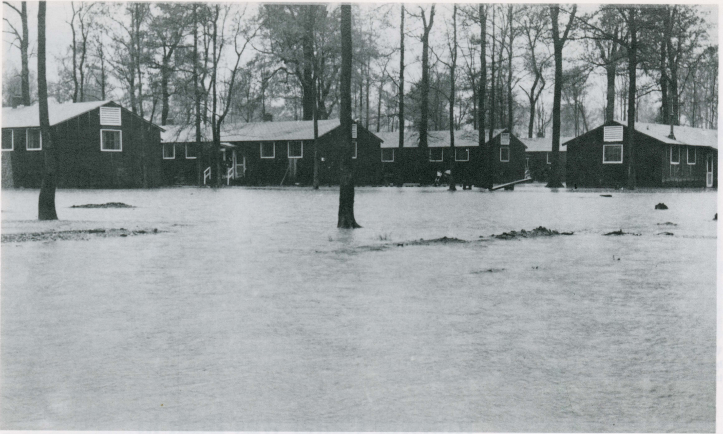
AND WHEN IT RAINS . . . Built in the delta area, the back portion of the camp was often flooded whenever an Arkansas downpour occurred.
