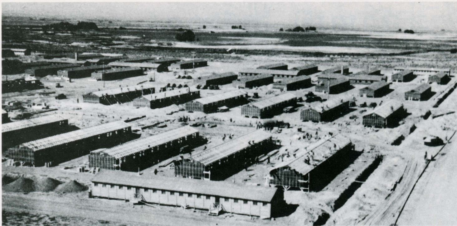
BIRD'S EYE VIEW —Rohwer concentration camp under construction during 1942. The camp began construction in July, 1942 and was completed in January the following year, which was three months after the
