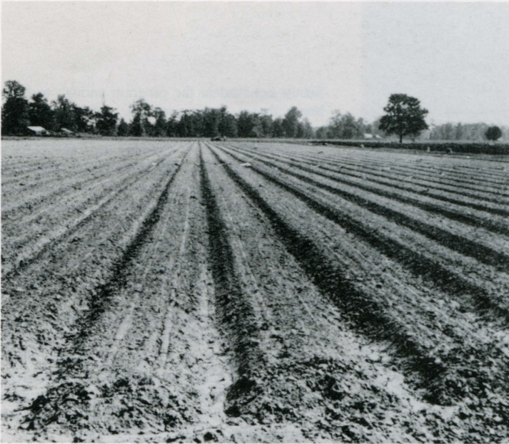
ROHWER FARM —Ready for planting are cultivated rows after internees had cleared and drained the land.
