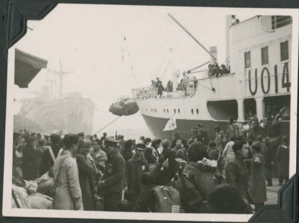
No. 2 GANGPLANK... HAUL BAGGAGES, UNLOADING OF-
