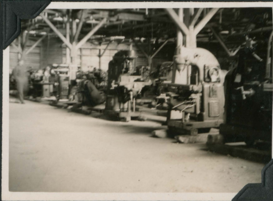
MORE MACHINERY LISTED FOR REPARATION
