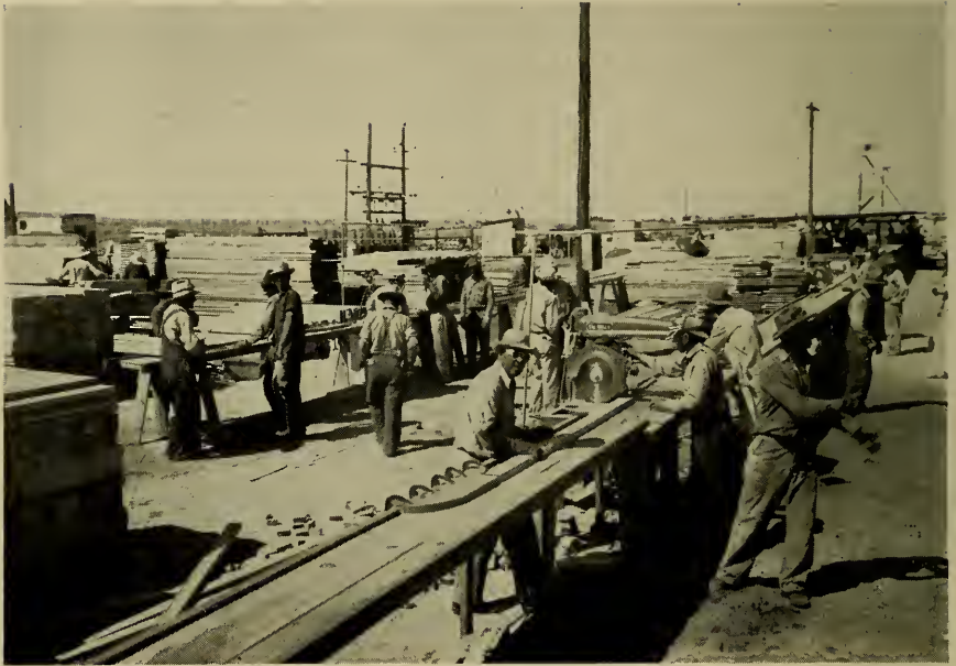
FIGURE 142: While the evacuation program was under way placing persons of Japanese ancestry in Assembly Centers, construction of War Relocation Centers was begun by Army Engineers. Construction operations at Heart Mountain Relocation Center, near Cody, Wyoming.
