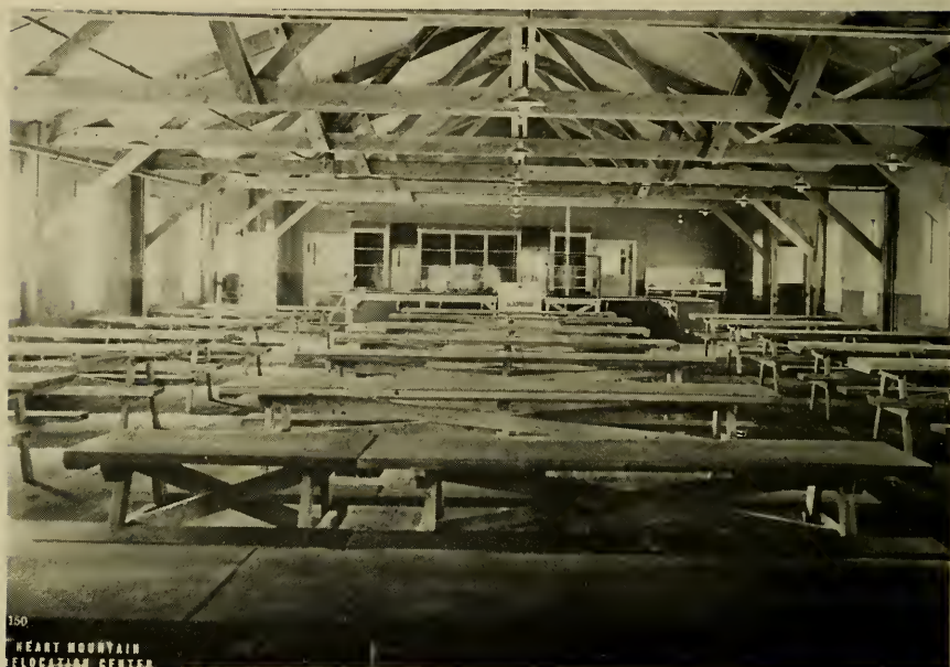
FIGURE 146: Typical mess hall in a Relocation Center hospital unit is completed by Army Engineers.
