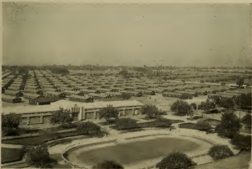
FIGURE 2: A portion of the completed Santa Anita (California) Assembly Center, situated within the world famous race track at Arcadia, California. This was the largest of all Assembly Centers. Nearly 19,000 persons were lodged here.
