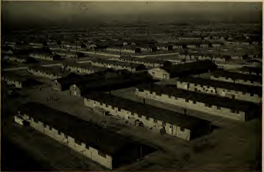
FIGURE 145: Panorama of Granada Relocation Center, Amache, Colorado, showing in the foreground a typical barracks unit consisting of 12 six-room apartment barracks buildings, a recreation hall, laundry and bathhouse, and the mess hall, constructed by Army Engineers. The Center is made up of 30 such blocks, complemented by hospital buildings, administrative office buildings, living quarters, general warehouse structures and Military Police quarters.
