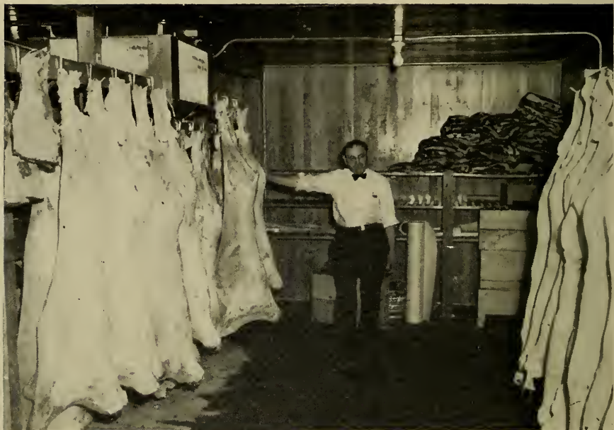
FIGURE 42: A scene in the meat storage room at Santa Anita (California) Assembly Center. Evacuees received a balanced ration, which included fresh meat, vegetables and fruits. Refrigeration facilities were provided at all Centers.
