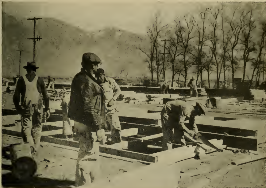
FIGURE 1: An early construction scene at Manzanar Reception Center, in Owens Valley, Inyo County, California. This was the first of a series of Centers constructed by the Army, and later became a Relocation Center under the War Relocation Authority.
