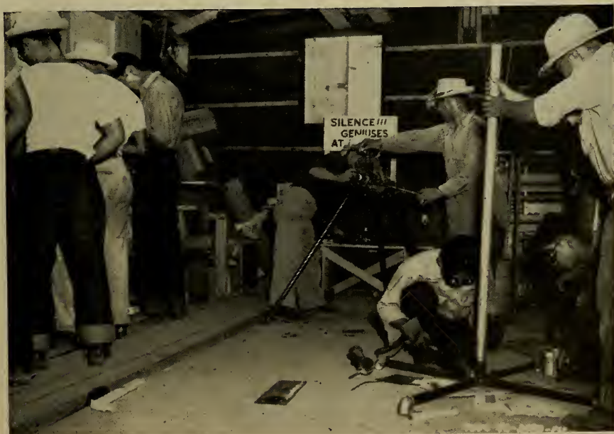
FIGURE 130: Diversified outlets for mechanical skills provided work with pay for many evacuees in the Assembly Centers. A group of mechanics welding an upright in the plumbing shop at Fresno (California) Assembly Center.
