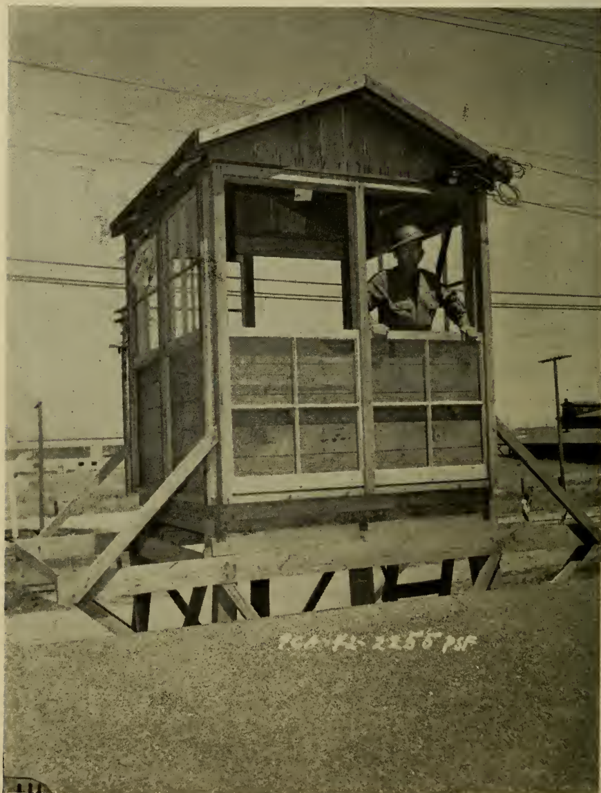
FIGURE 23: Guard on duty in watch tower at Tanforan (California) Assembly Center. The Military Police were responsible for the external security of the Assembly Centers. In addition to details of Military Police assigned to the external boundaries of the Centers, guard towers were erected at strategic points and a watch kept for fires or other dangers.
