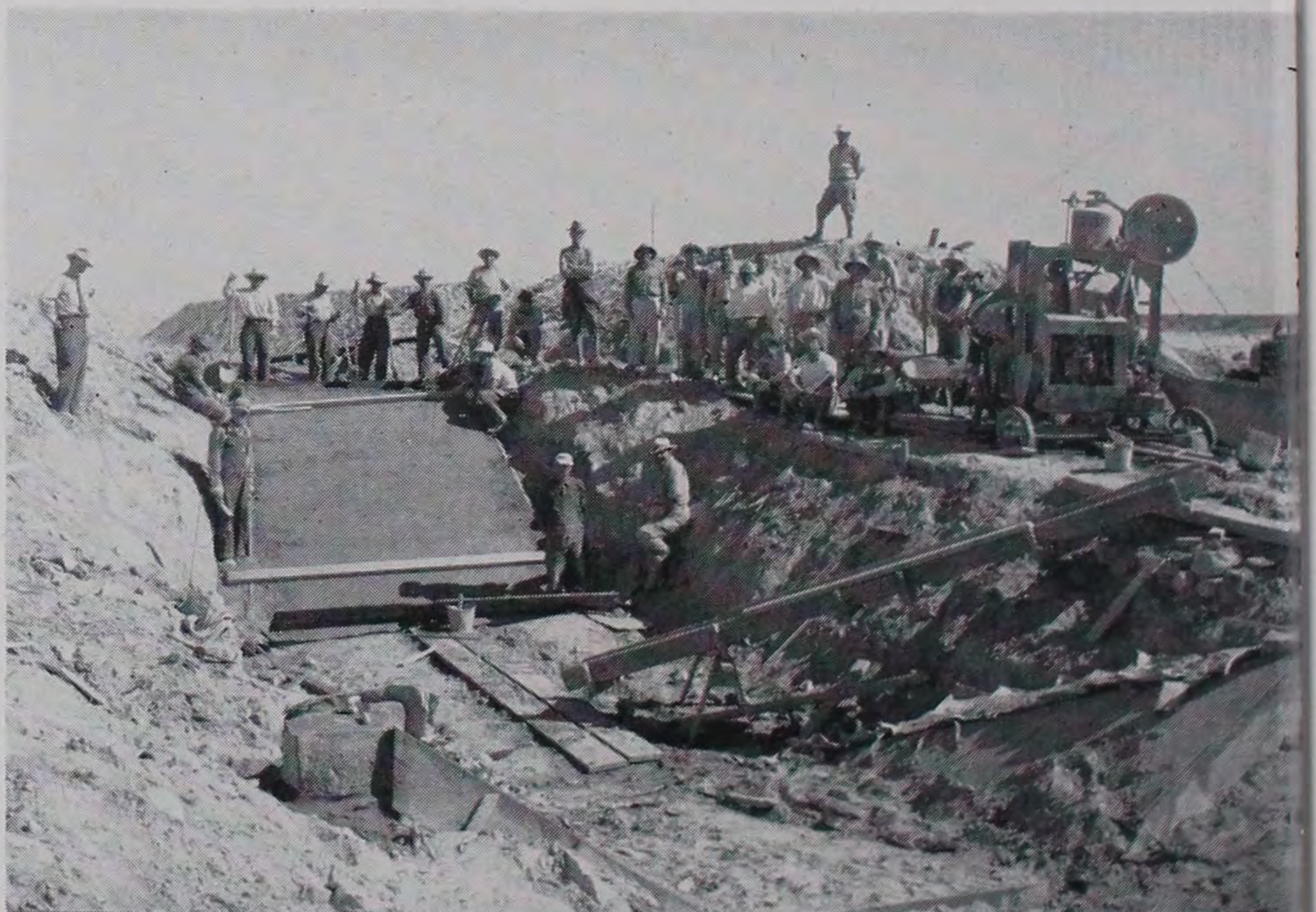
CONSTRUCTING A DROP
