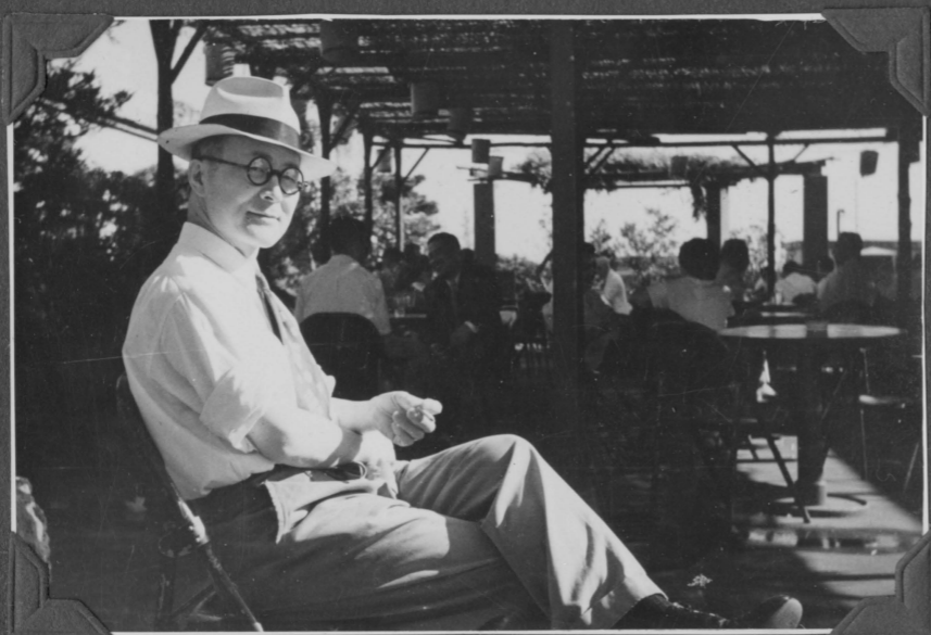
Roof Garden Marunouchi Bldg., Tokyo September 6, 1952 (Courtesy of Dr. Herman Gray)
