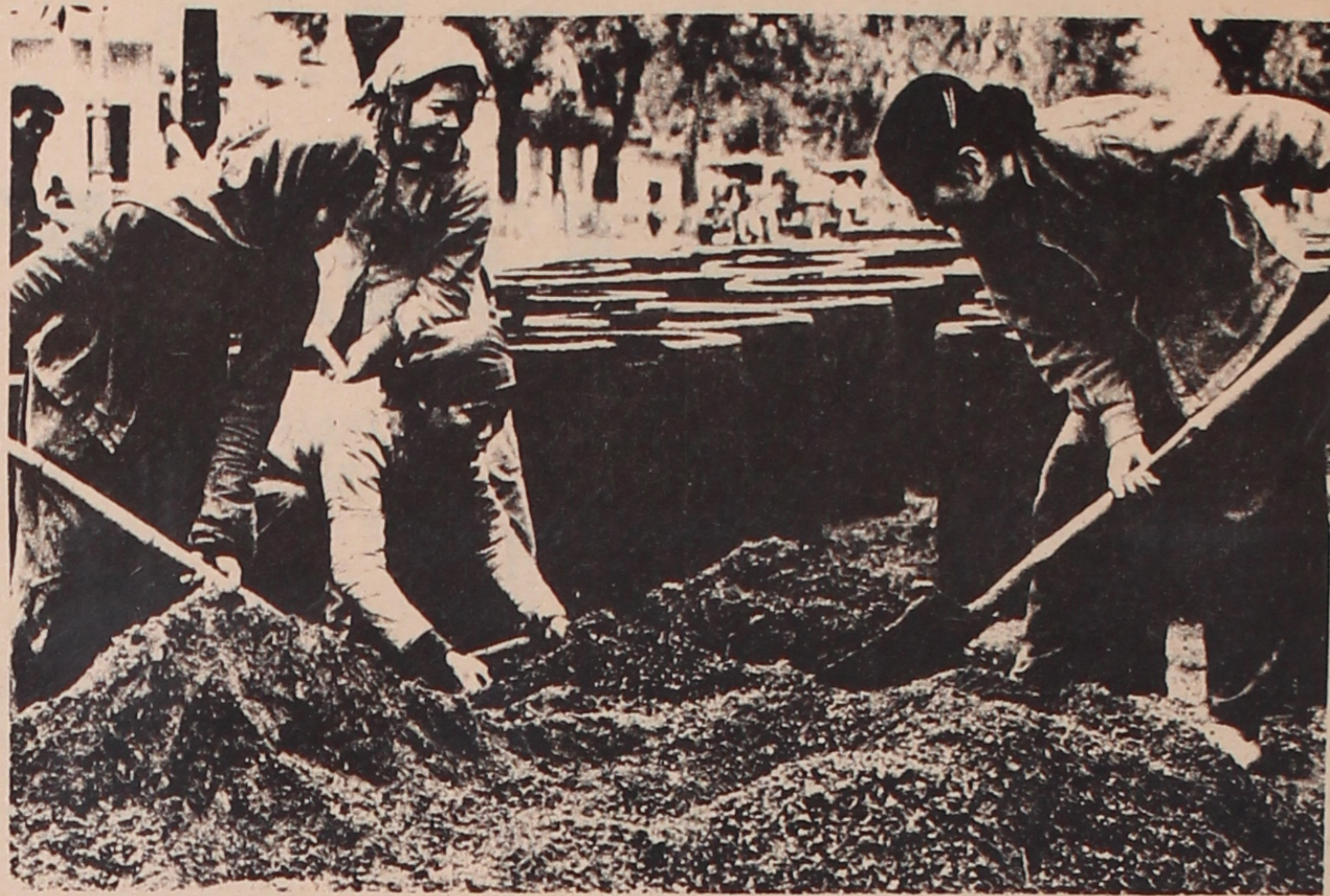
Women at work manufacturing individual air-raid shelters on one of the main streets of Hanoi. The shelters are made of concrete cylinders that are embedded in the ground. Each holds one person.
