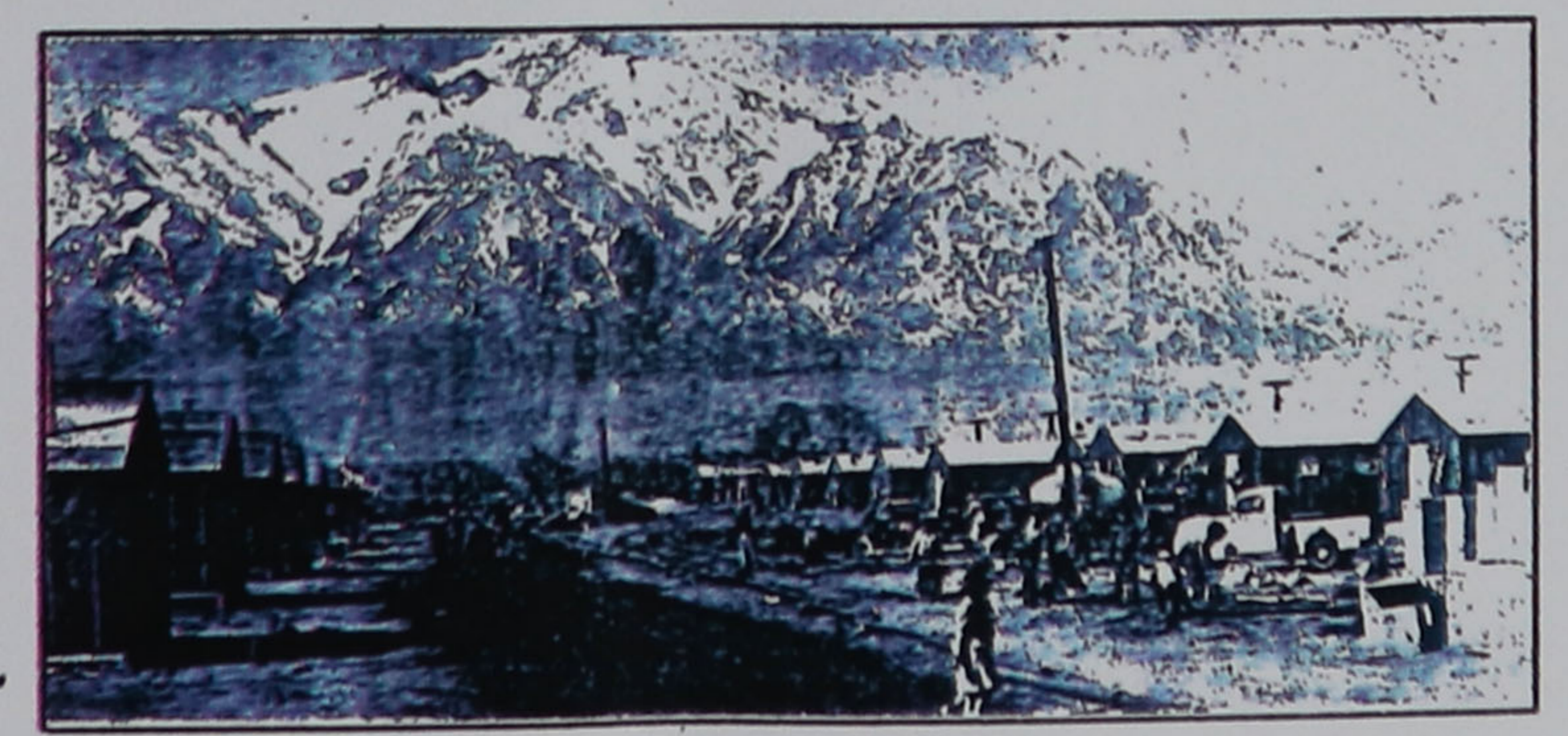
Familiar view An early photo of Manzanar with construction still in process. Along this road, men laid down pipes. The peak is Mt. Williamson (14,373 ft.)
