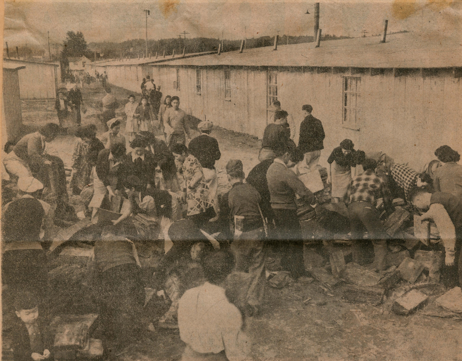
Everybody works at the Puyallup camp for evacuated Japanese. Since all the camp's stoves are wood burners, every family has developed a tremendous interest in wood deliveries made at street ends
