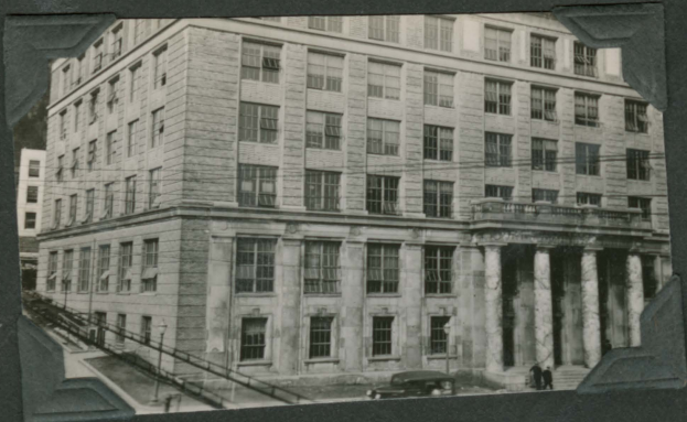
Capital Building Juneau
