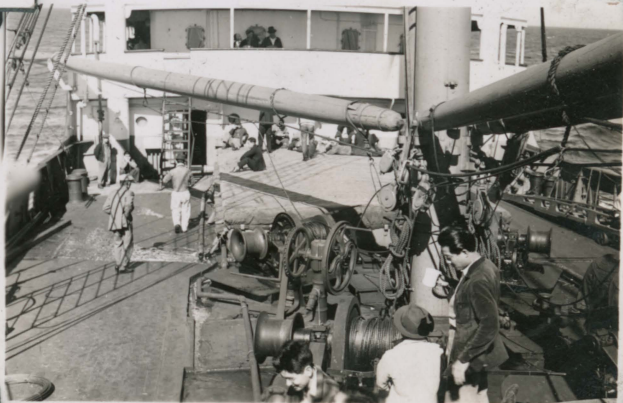
Hoisting on deck
