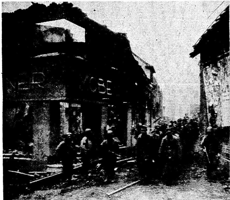
ON THE MARCH—Germans captured in a Siegfried Line pillbox by United States First Army troops are marched into Palenberg, Germany, past buildings that show evidence of the heavy fighting on German soil. Photo by Harry Harris, Associated Press photographer with the wartime still-picture pool.
