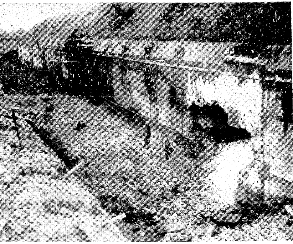
TNT IN TRUCK DID IT—Two American soldiers examine a hole in the wall of a German-held fort near Metz, France, after United States Army engineers had loaded a German half-truck with TNT and rolled it into the side of the structure. Eighty-two Germans surrendered to an American Infantry company after the blast.—A. P. wirephoto from United States Signal Corps.
