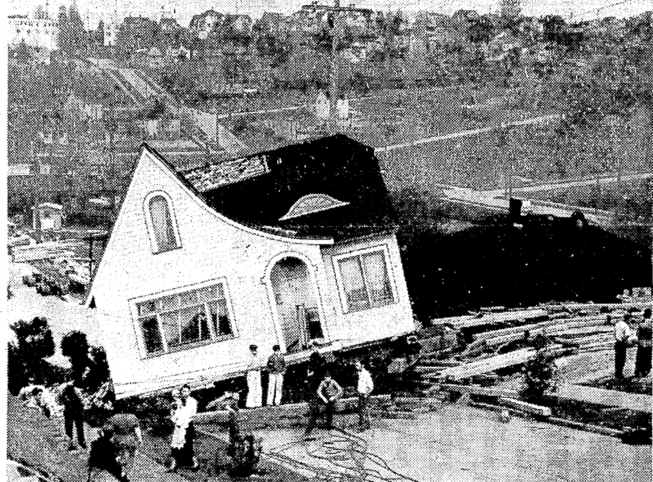
Richard Gregory, construction company employe who built this house three years ago at 2453 Day St., learned yesterday that his home has a mind of its own. At the start of a four-block trip to a new location in Irving Street, the house slipped from cables and "sat down" in Day Street. It stayed there last night and resumed its journey today. The house is being moved from an area being cleared for the Lake Washington Pontoon Bridge approach.
