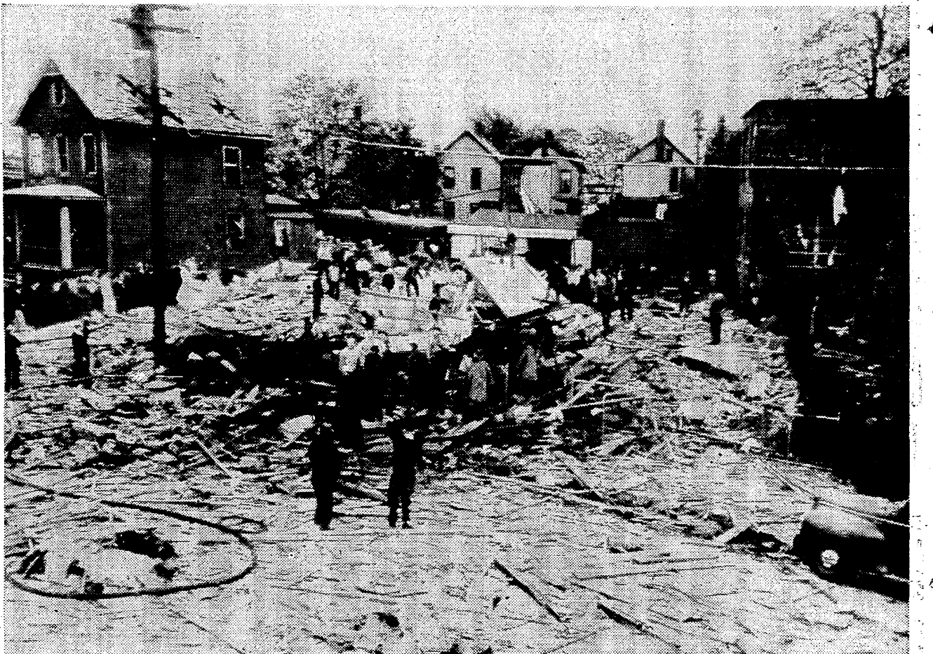
IN NEW BRUNSWICK, N. J., YESTERDAY One person was killed and at least eight were injured when an explosion leveled a two-story brick building housing a chemical plant. Here is a general view of the wreckage showing also damage to windows and roof of house at left.—A. P. wirephoto.
