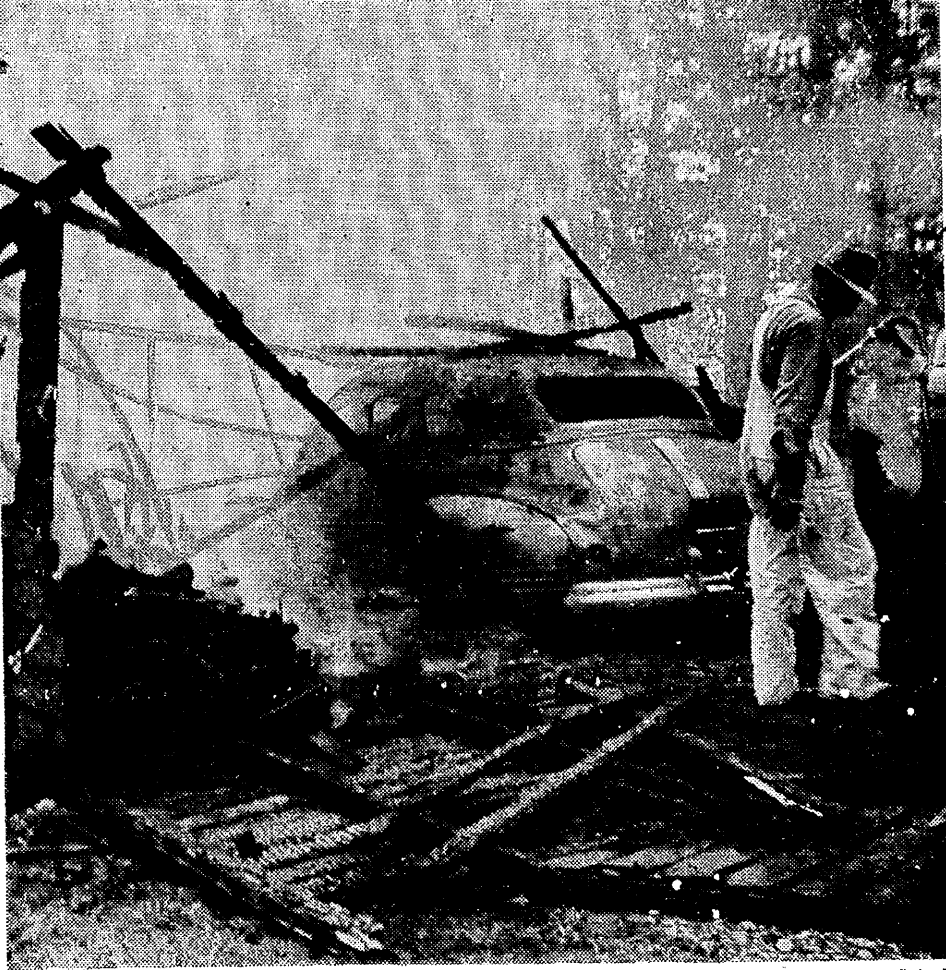
Herman E. Hanson, 11528 Roosevelt Way, left his 1942 automobile at home yesterday and took a bus to save gasoline. But a few hours after he left, fire of undetermined origin burned the garage to the ground and destroyed the automobile. Now Hanson will be taking the bus every morning.—Photo by Robert Ford, 1312 N. 43rd St., who receives $3 from The Times.
