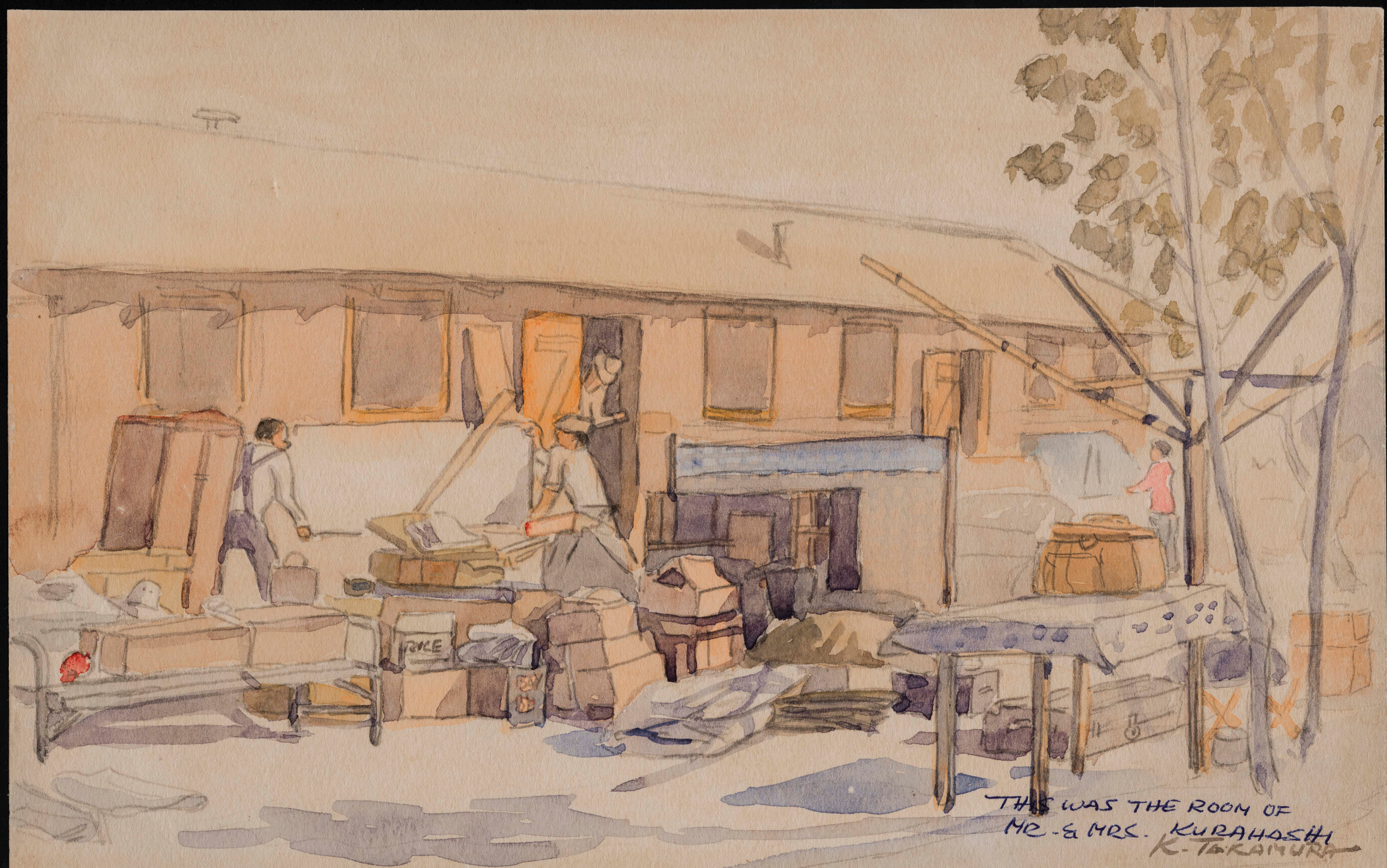
RESIDENTS INSTALLED PLASTER BOARDS INSIDE BARRACKS.
