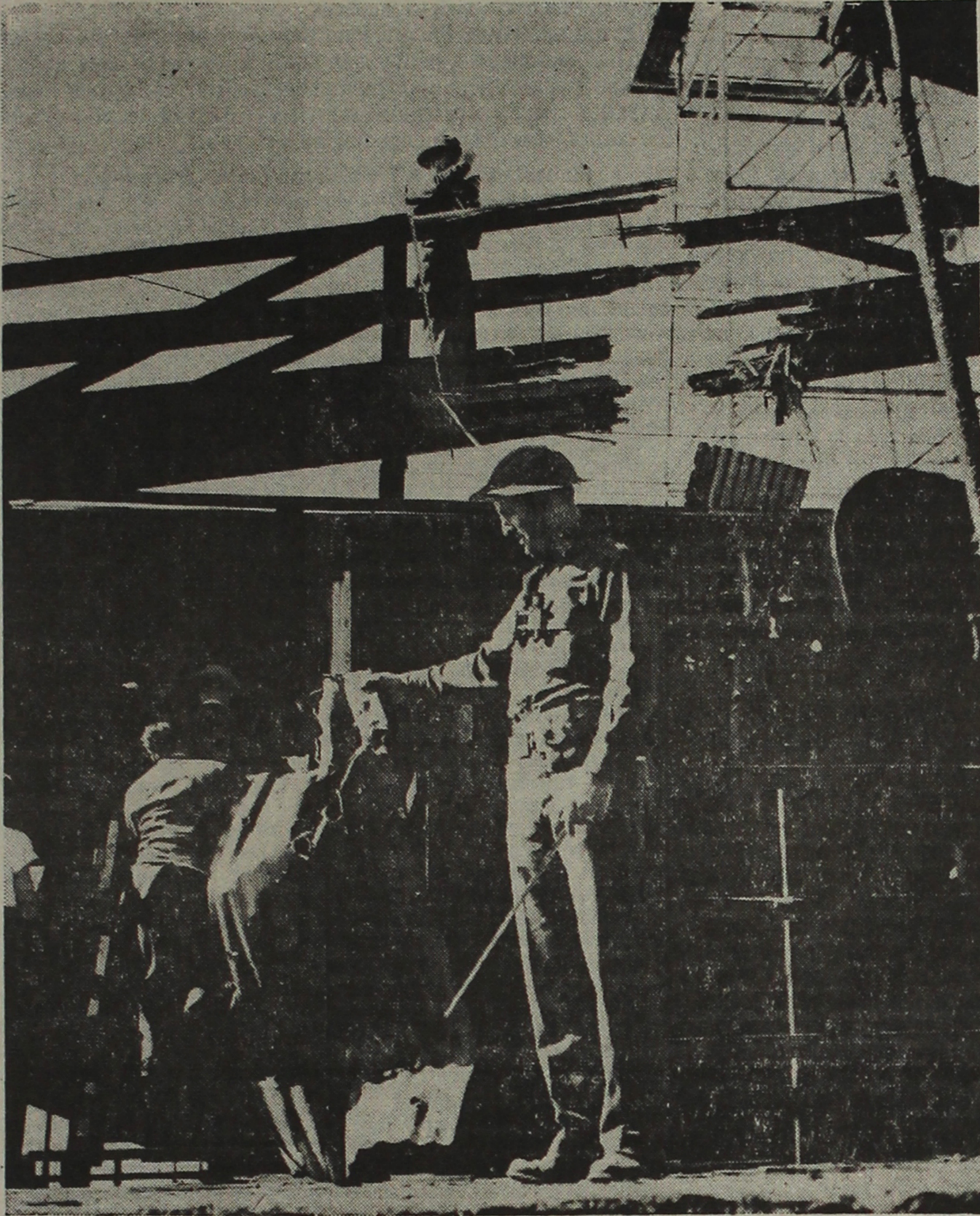
SUBMARINE DAMAGE from the 1942 attack was confined to a splintered catwalk on Luton Bell No. 17 oil well and shrapnel-riddled sheet iron in the vicinity. The officer shown inspecting the damage, Maj. Bernard Hagen, was later injured while defusing a dud shell found on the premises and received the first Purple Heart medal issued for enemy wounds suffered on the American continent during World War II.
