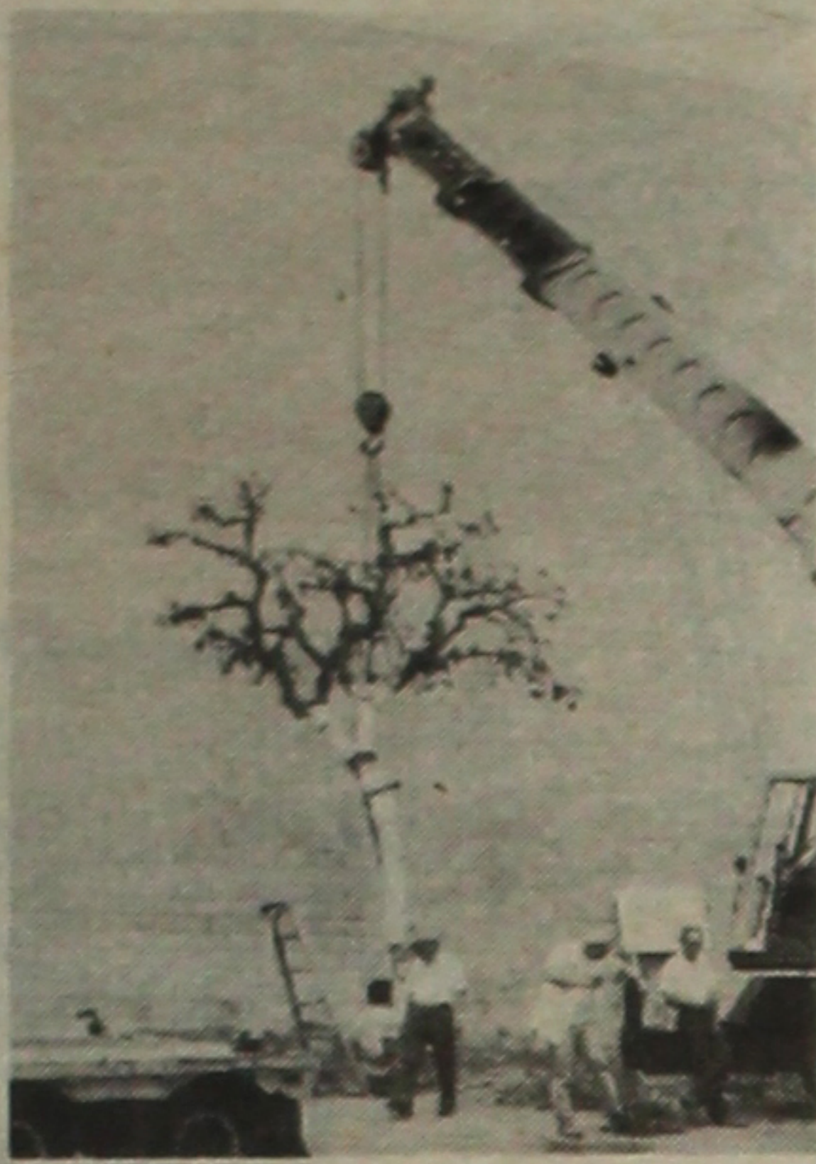
Kashu Mainichi UPROOTING—Workers use crane to save 100-year-old tree.
