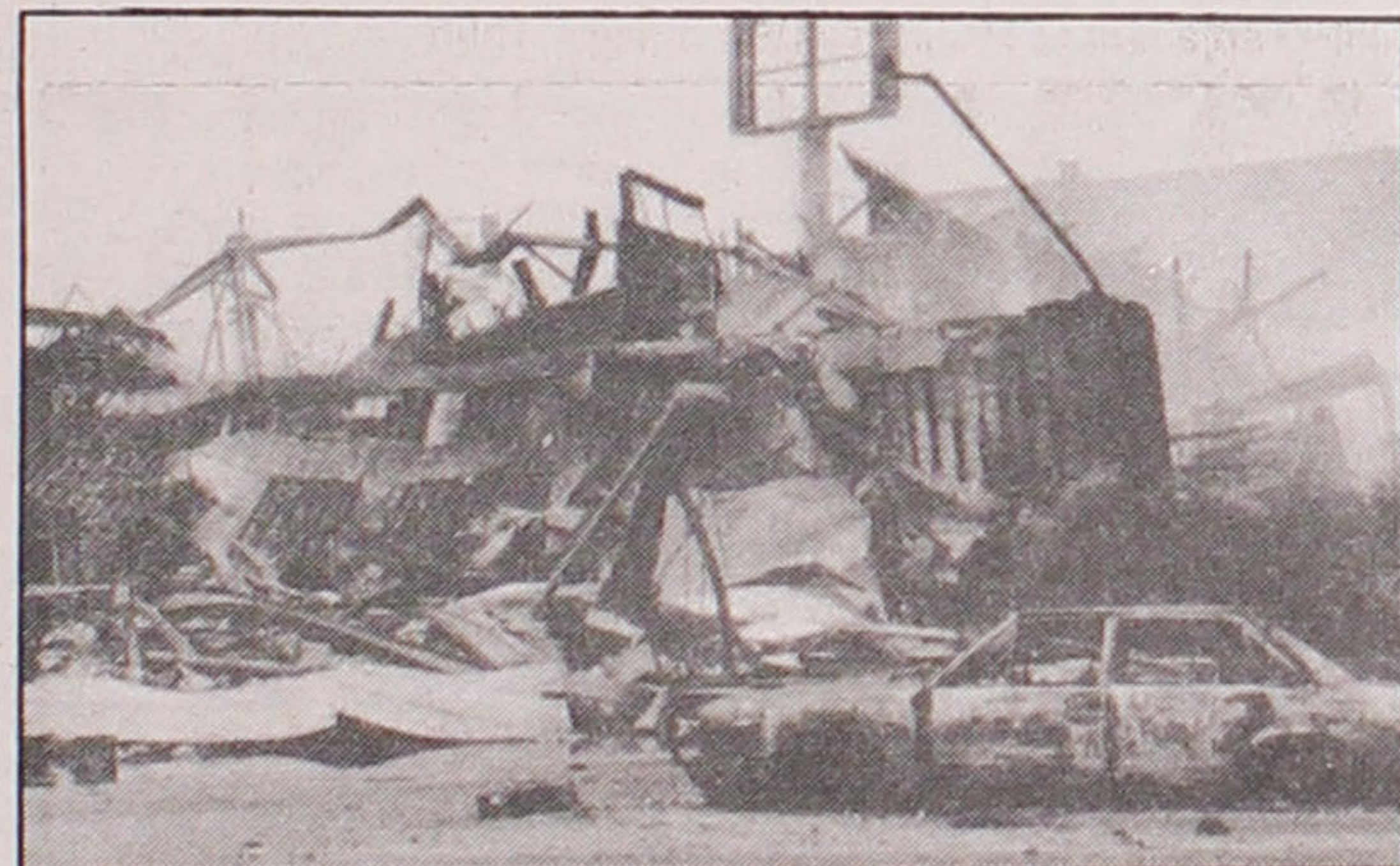
DEVASTATION —Totally-gutted are two Crenshaw Square stores and Crenshaw Medical Center (once housing Nisei physicians). Wall at right is the Sumitomo Bank of California.
